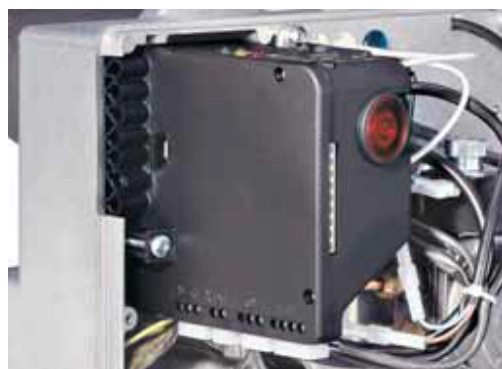
Control box fitted with ignition transformer
